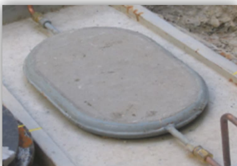
Figure 4: Filling the central volume using a resin mortar
