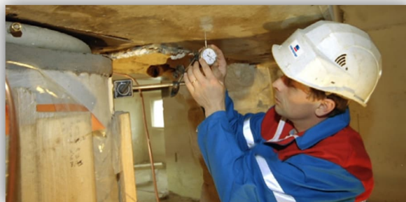
Figure 6: building lifting & displacement monitoring
